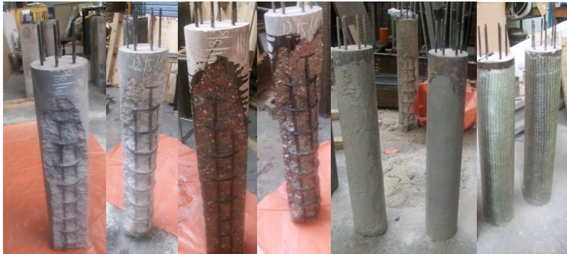
(a) (b) (c) (d) Fig.6: Spalled columns before repairing (a-b) after repairing with epoxy resin mortar© and GFRP (d)
