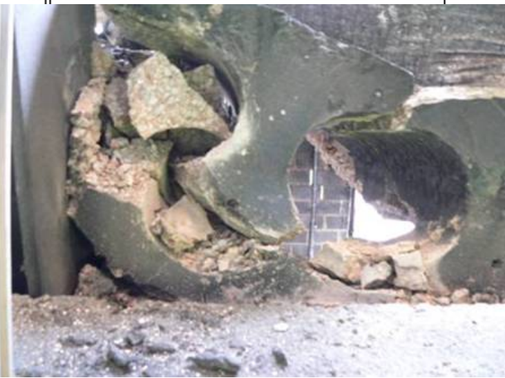
Evidence of a lateral compressive strip forming enhancing flexural and shear capacity
