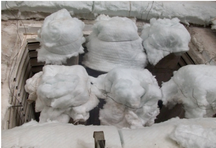
Fig.5: Columns before heating
