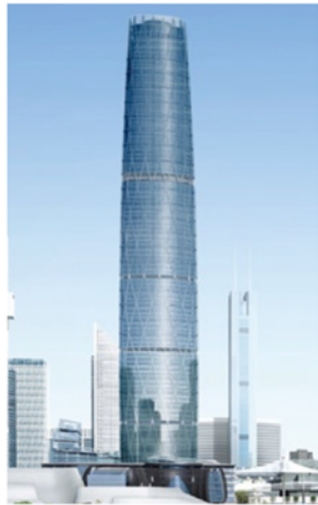
Guangzhou TV Tower 2010 610m
